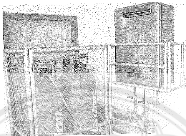
Figure 13 The Rainnai Infinity 32 and the LPG as the auxiliary heat sources
