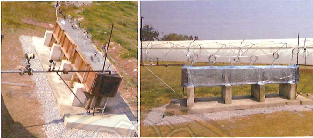
Figure 21 Install sensors and concrete materials
